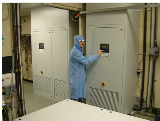
Figure 2. Photo of new air conditioning units after installation.
